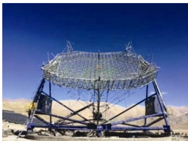
Figure 5. The status of the telescope installation at Hanle in December 2016. The two instrumentation shelters are mounted on the alidade structure. The solar photovoltaic panels deployed for providing electric power to the telescope on the left of the photograph.
